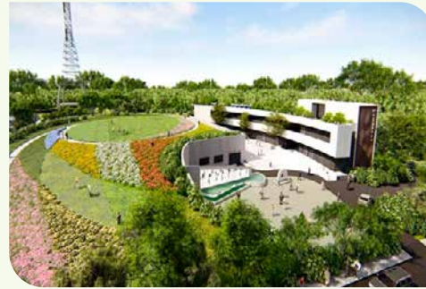
▲ Figure 5-7 Taoyuan Metro Station A7 Water Recycling Center
